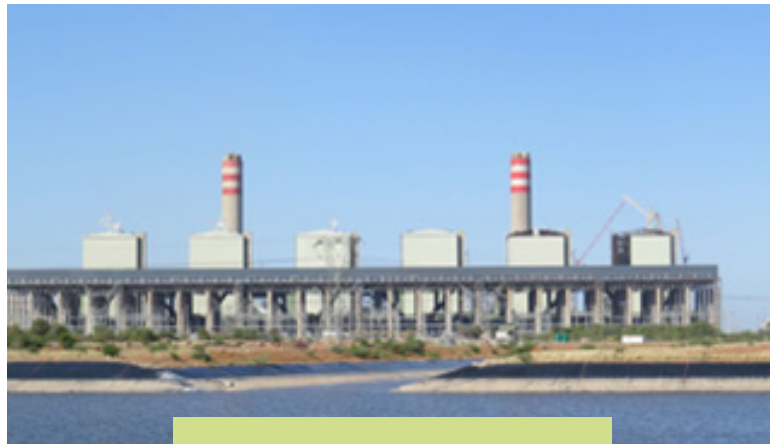
Kusile power station © Eskom
